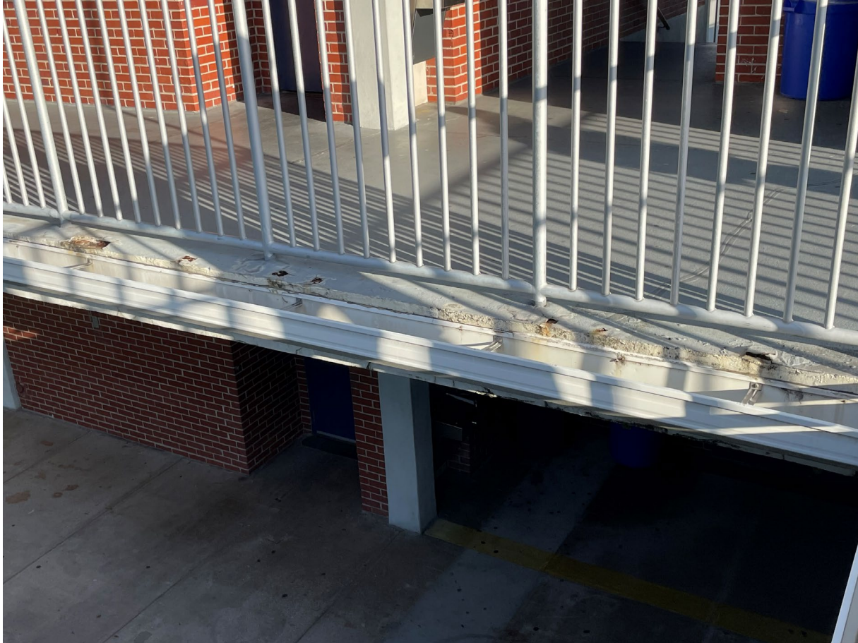
Examples of Concrete Spalling at West Shore Jr./Sr. High School
