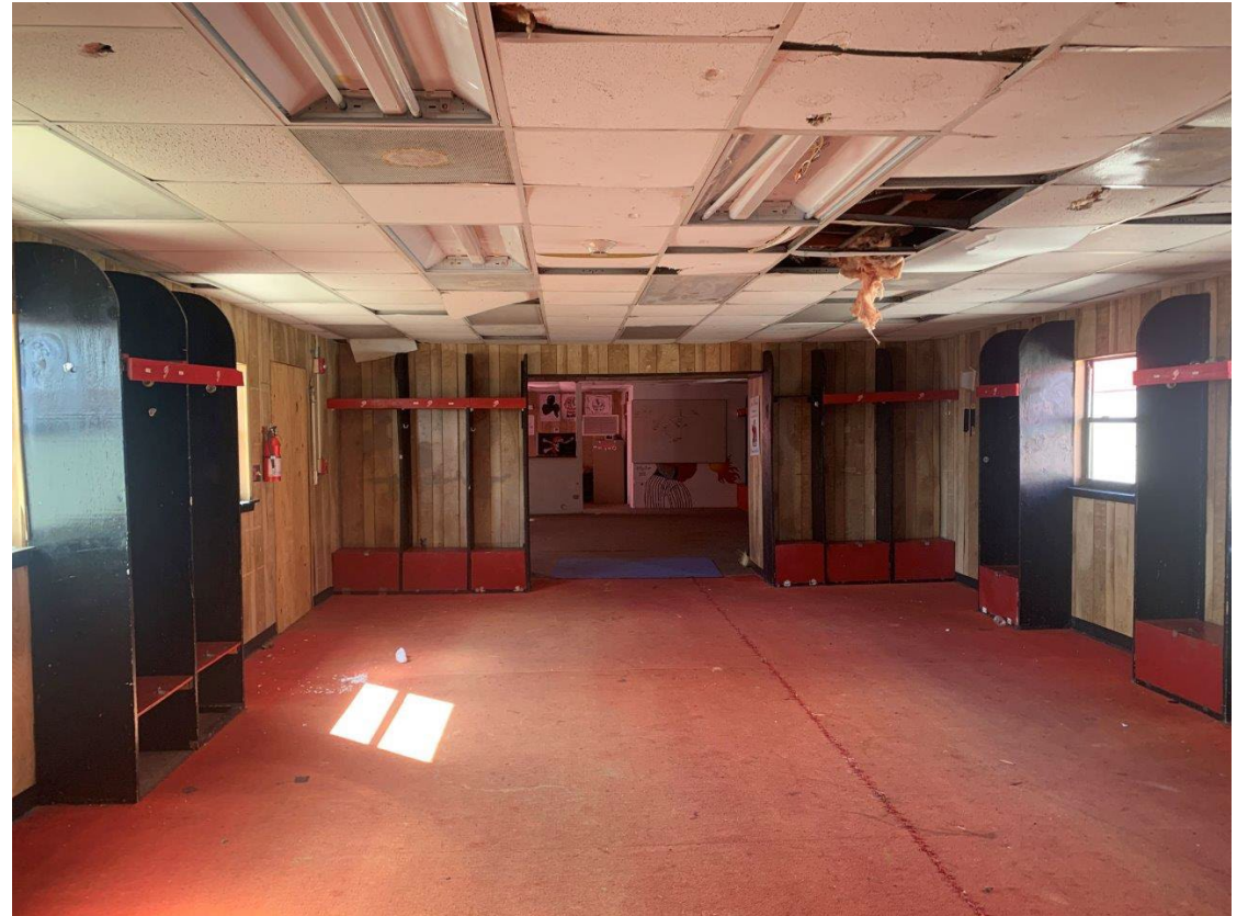
Portable N942 – Recommended for Demolition
